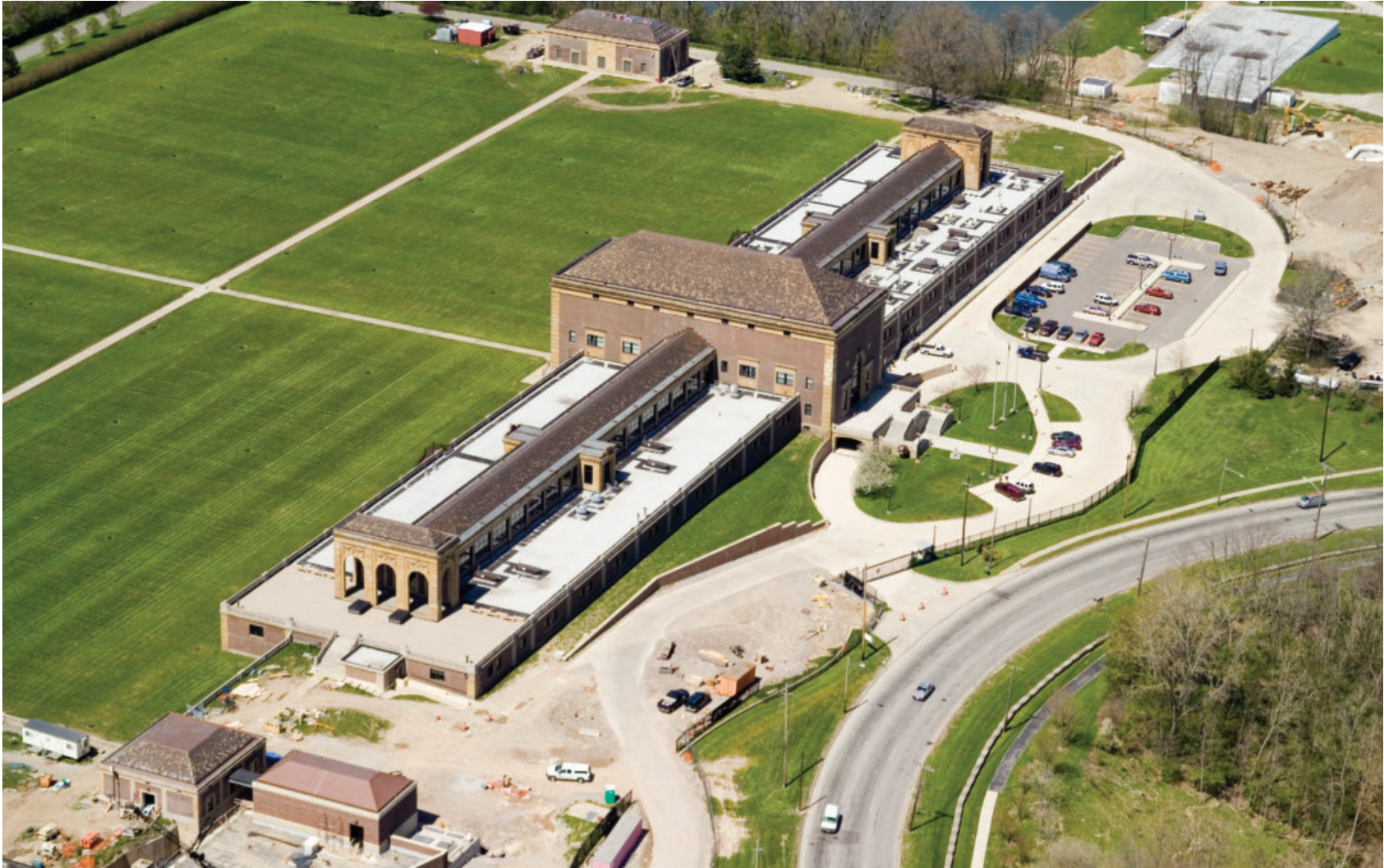
Cleveland Water Department, Baldwin Water Plant Expansion Cleveland, Ohio
