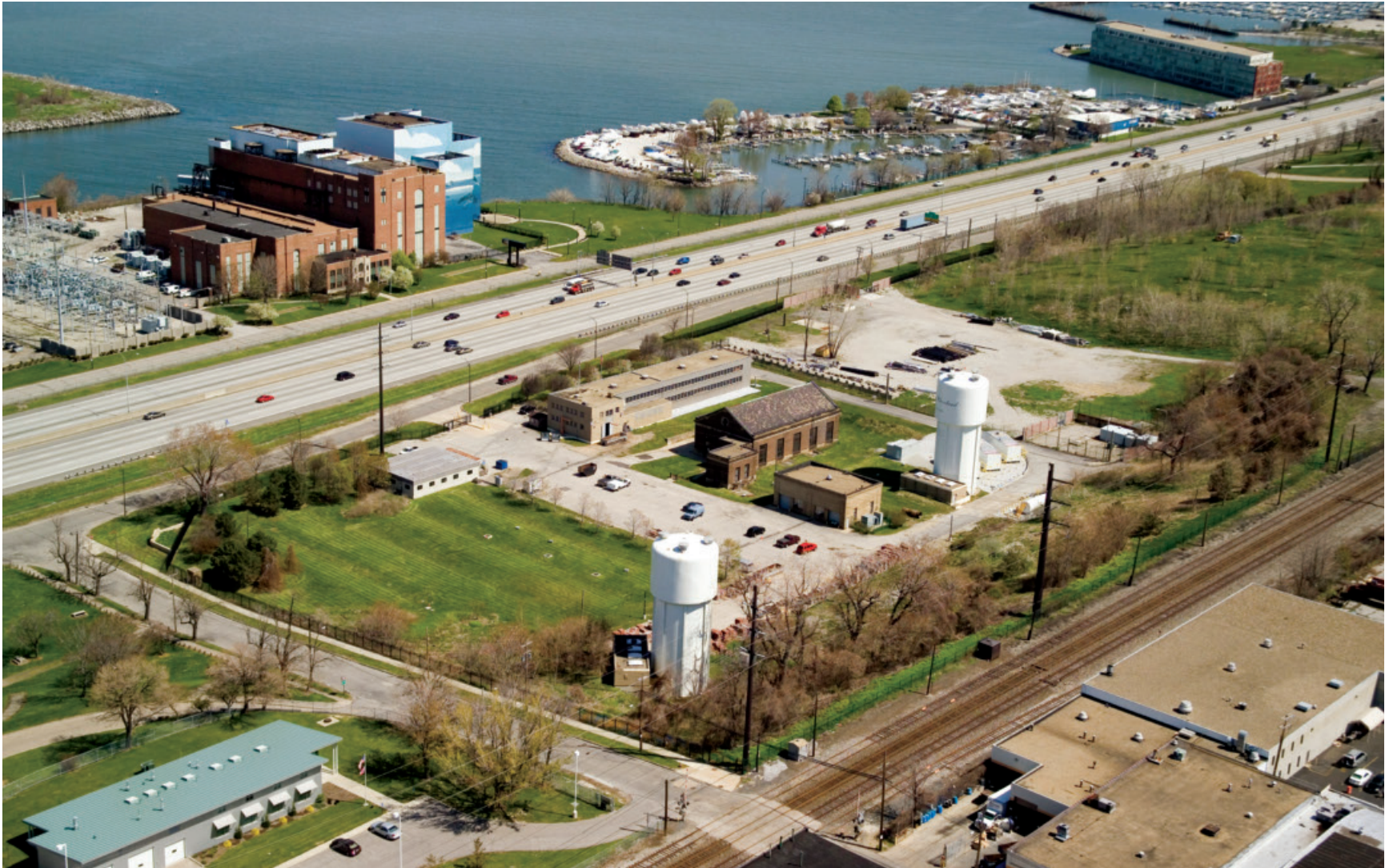
Cleveland Water Department, Kirtland Water Plant Expansion Cleveland, Ohio
