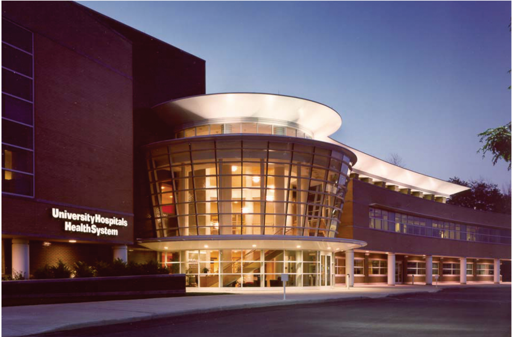
University Hospitals Westlake Facility, Westlake, Ohio
