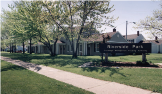
Cuyahoga Metropolitan Housing Authority Riverside Estates Comprehensive Renovation Cleveland, Ohio
