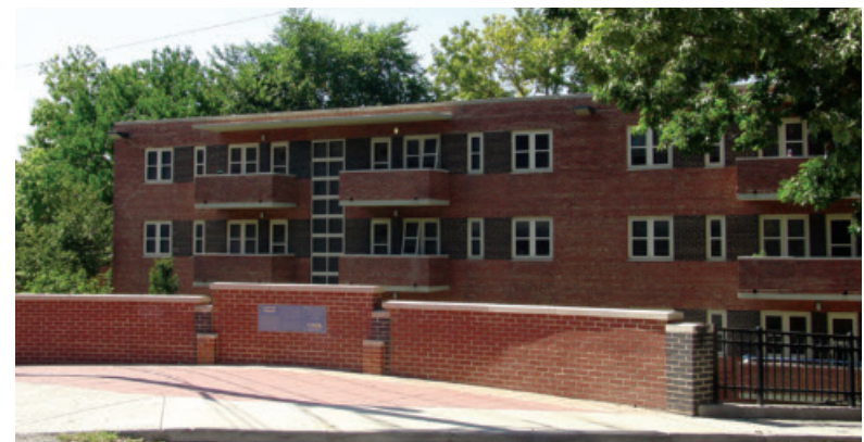
Cuyahoga Metropolitan Housing Authority Lakeview Estates Cleveland, Ohio
