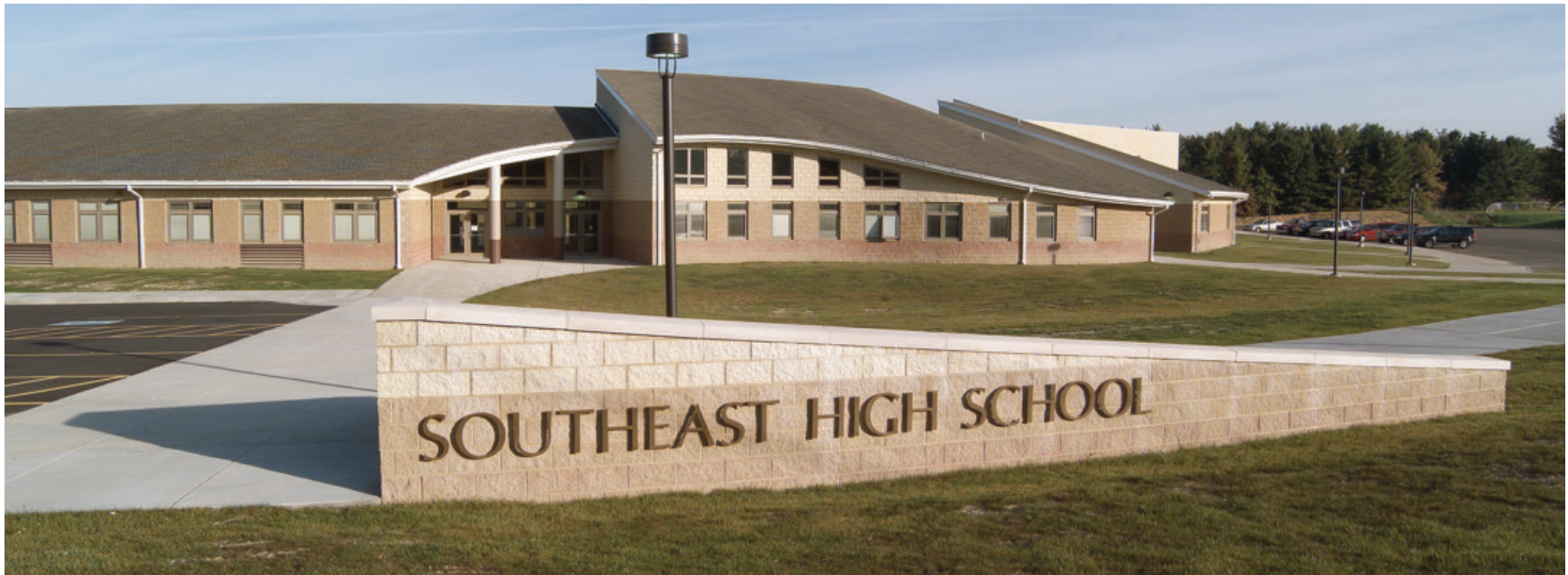
Southeast High School, Southeast Local School District Ravenna, Ohio
